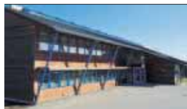
STEMA/PEDAX Headquarters – Denmark
